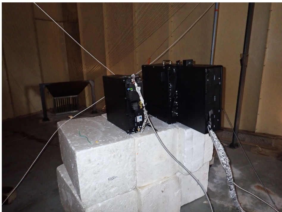
Test Setup of EG4 LL100Ah 48V Server Rack (Serial No. SC2022101794) and EG4 18kPV Hybrid Inverter (Serial No. 3464660222) on Y Axis
