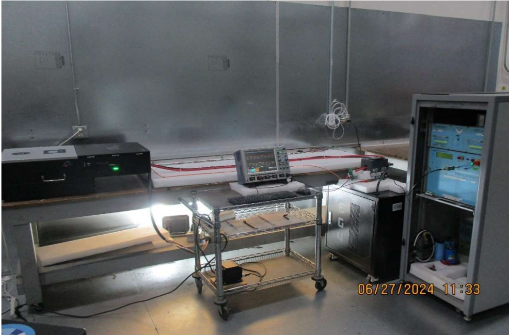
Test Setup for CS117, General Waveform #2 & #3 Test Setup for Battery Rack Mount
